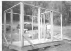
Volunteers from Colorado Springs constructed a shower unit at Elk Creek Ranch
